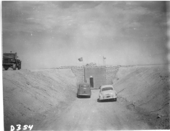
Revetment station #228, for data recording, project 8.12a, 6 May 1953
